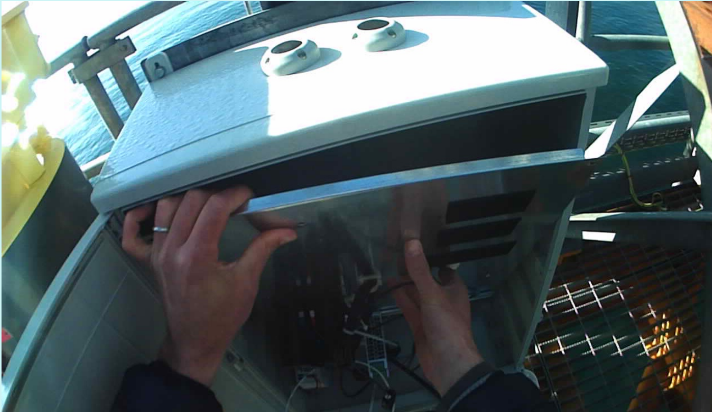
Fitting the metal plate with electrical components pre-assembled
